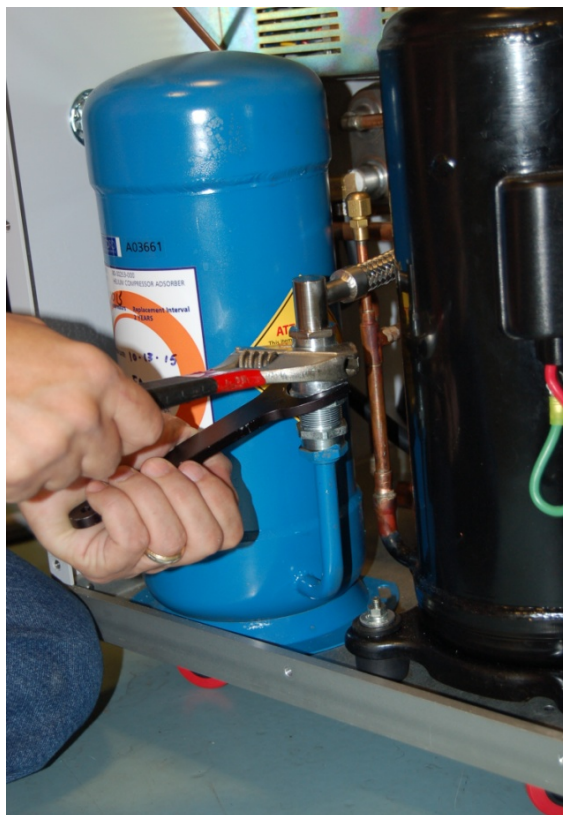
Figure 7 – Adsorber Aeroquip OMS Supply Line Removal
